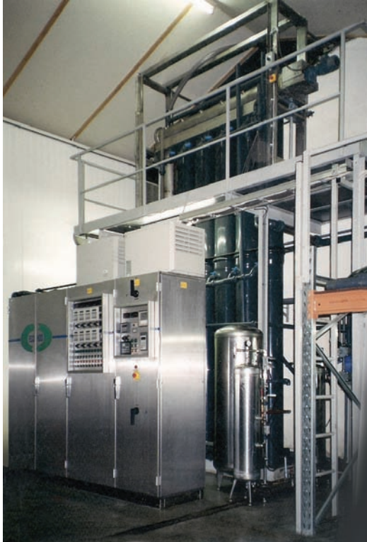
The small MUST Water Purifier produces drinking water even from cow manure at a capacity of 44 000 m 3 /year.
