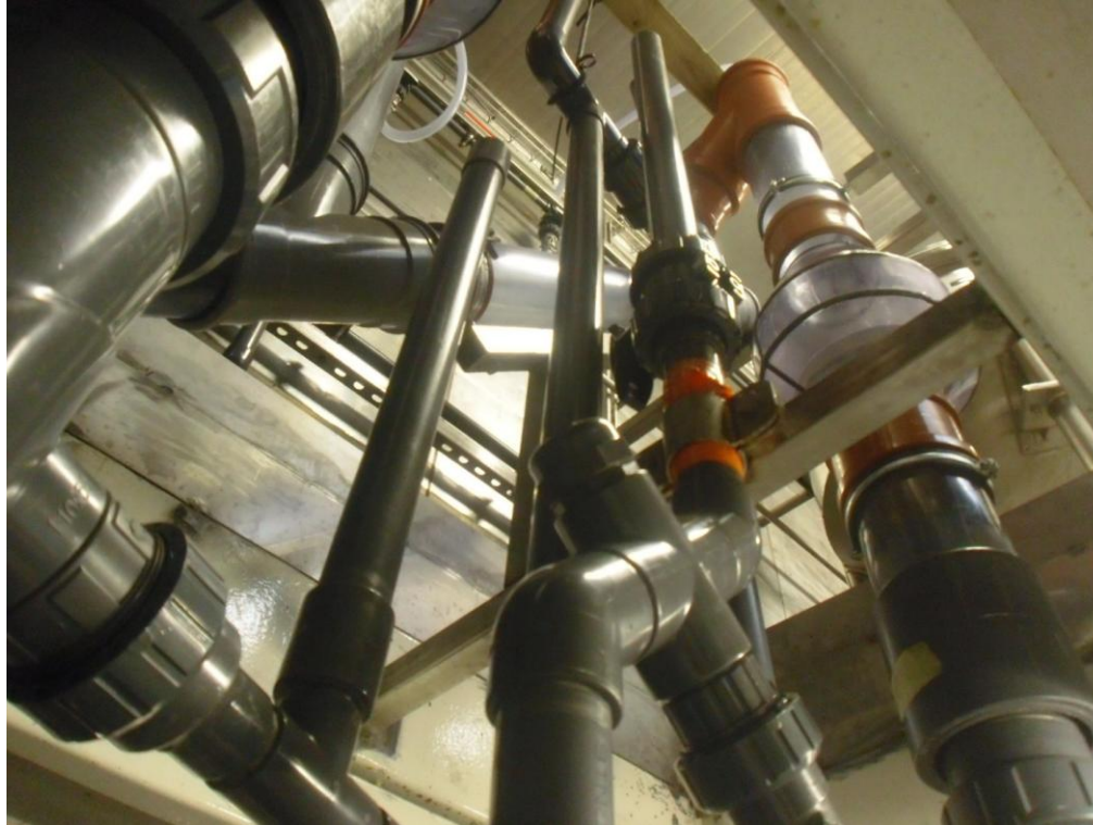
Picture 6: The floc separation tower extends above the MUST cell. The dewatering floc will glide down along the vertical dropping tube in the upper center of the picture. The purified water will be collected from the bottom of the tower in the bottom right corner of the picture.
