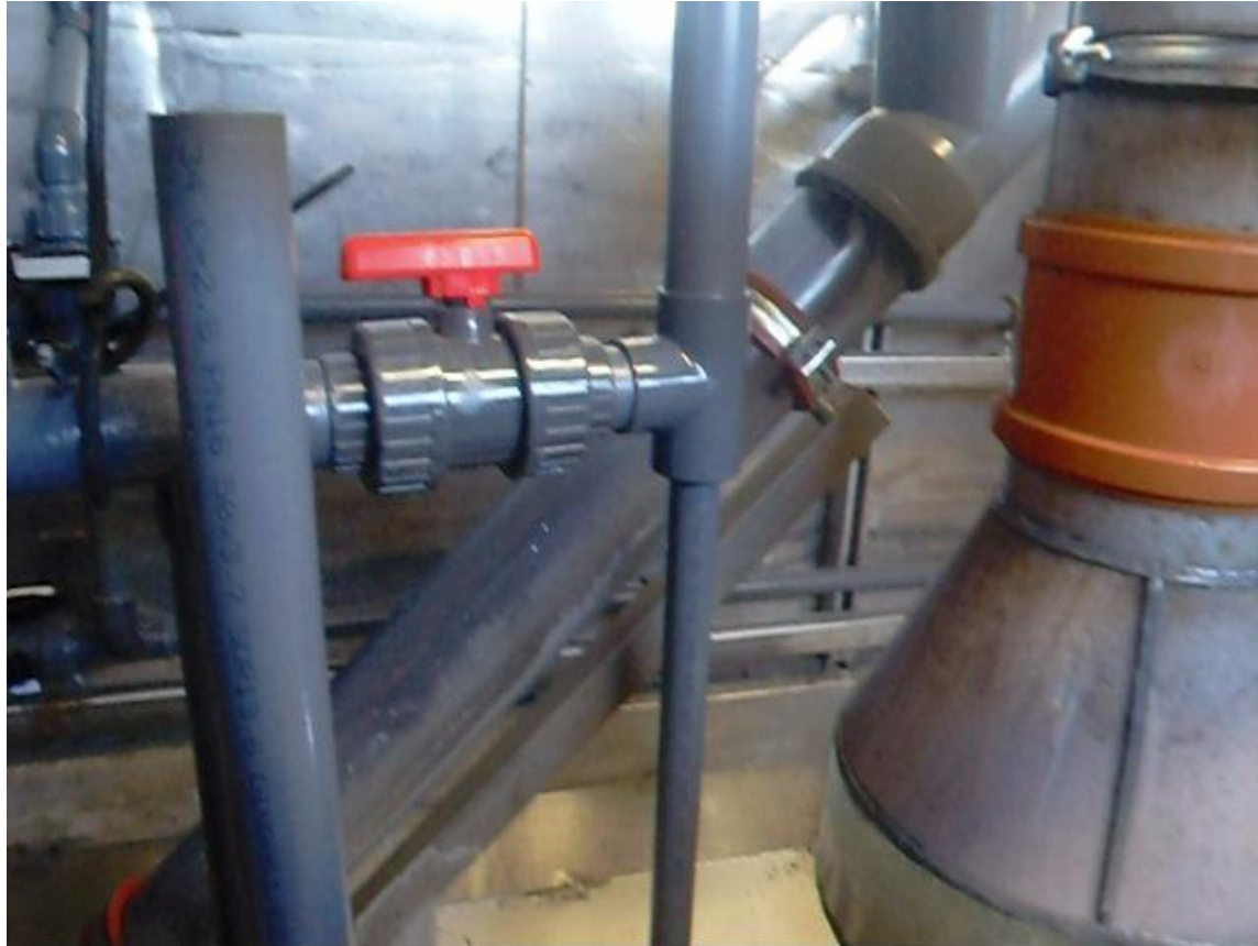
Picture 9: Video clip: Pollutants in the floc are continuously removed upwards from the purified water, which flows downwards. Floc glides along the dropping pipe into a decanter for dewatering.
